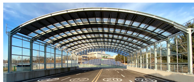
Soundproof Wall/Tunnel-integrated Photovoltaic System
